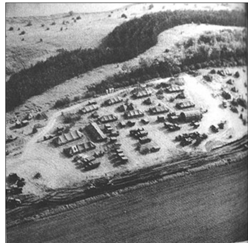
This is another helicopter photo looking down on the huge camp out and construction yard of all the guard equipment. Around 12 or more large tents are set up down below for mechanics fuel supply, first aid, mess hall and sleeping quarters. This big yard was right off the north and south county oil road, on the northside on the new lake access road. It was indeed a tent city out in the country. To this day that big flat area has stayed pretty open with only grass and small brush on it.
