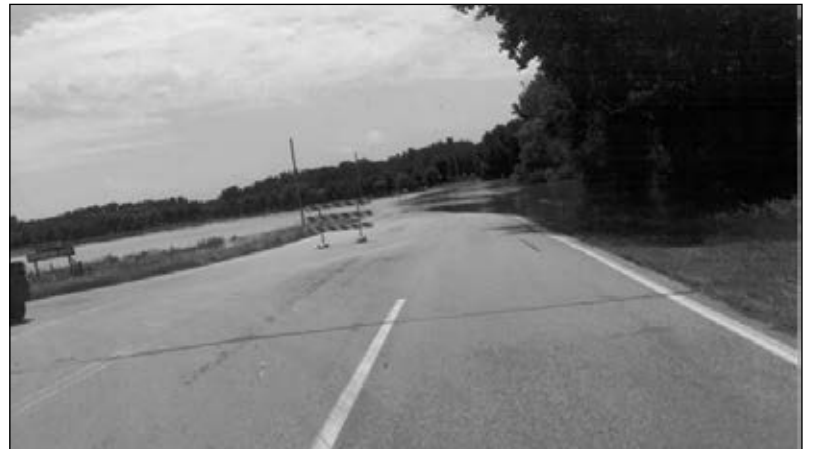
Going south of Canton on oil to Newton Hills, all traffic was barricaded off, as Beaver Creek was so high, it was even flowing over the top of the bridge rails and also the road into Beloit was blocked off, with a lot of water going over the highway making a loud rushing sound.
