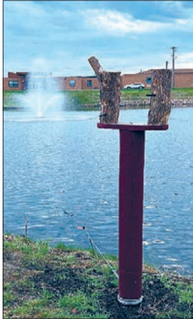
New aerator at Lake Ole with bird feeder atop the anchor
